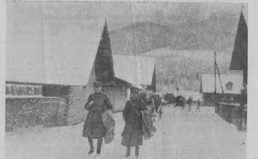
Ulica w Podspadach
